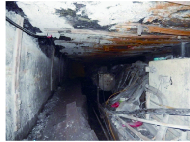
Fig. 9. Cutters developed at entry corners near the face.
