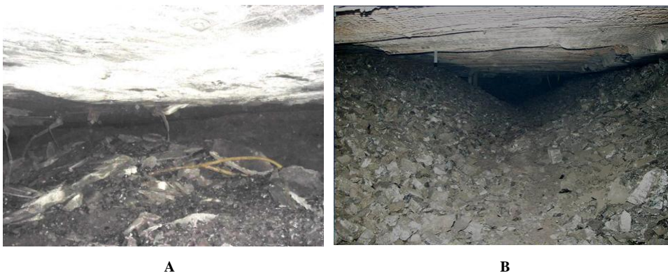
Fig. 9.1.1 Scenes of coal bumps. Note that the roof in both cases were undamaged and very often there is a gap between the roof and the top of the broken pillars (Boler et al., 1997; Hayduk, 1984; Newman, 2002)
