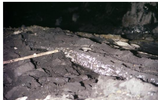
Fig. 10.6.3 Beam failure of floor. Left, Lueckenhoff et al., (1979). Right, Peng (2007)
