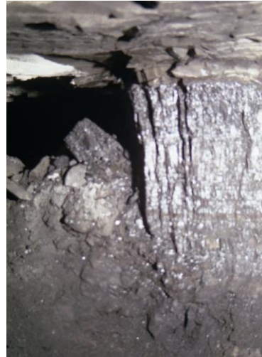
Fig. 10.6.2 Pillar punching of floor failure. Left, Lueckenhoff et al., (1979). Right, pillar punching accompanied by pillar spalling (Peng, 2007; Peng and Wang 1996)
