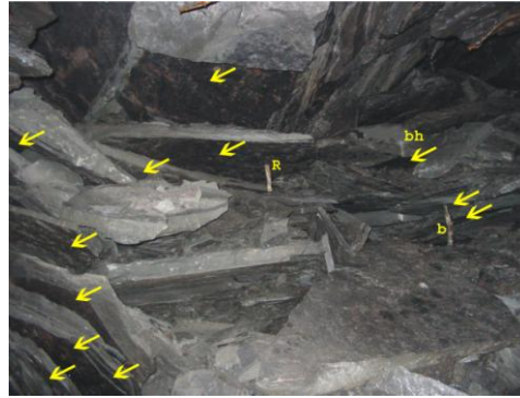
Fig. 10.2.4 Stack rocks. Arrows indicate thin film of carbonaceous materials. b is broken roof bolt, R is roof bolt, and bh is bolthole (Peng, 2007)
