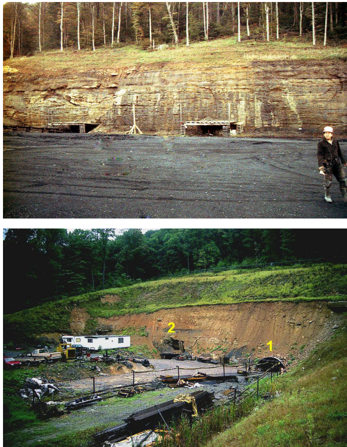
Fig. 14.1.1 Two examples of face-up highwalls in drift mines in Appalachia (Peng, 2007)
